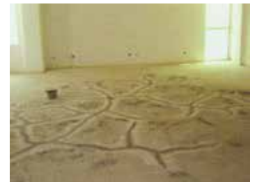
Repair cracks
